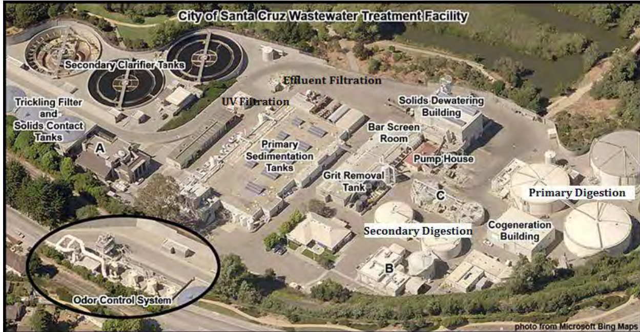
Figure 6-10. City of Santa Cruz Wastewater Treatment Facility
