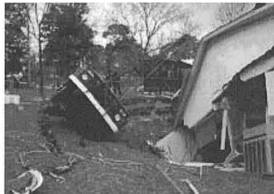
Fig. 29. Water well drilling near this Florida home triggered a sinkhole collapse beneath both the drill rig and the house.
